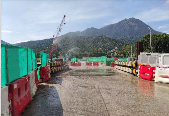
Water spraying via sprinklers at main access road
