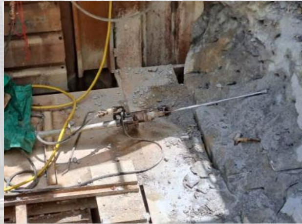
Concrete breaking by quieter method (Rock Splitter)
