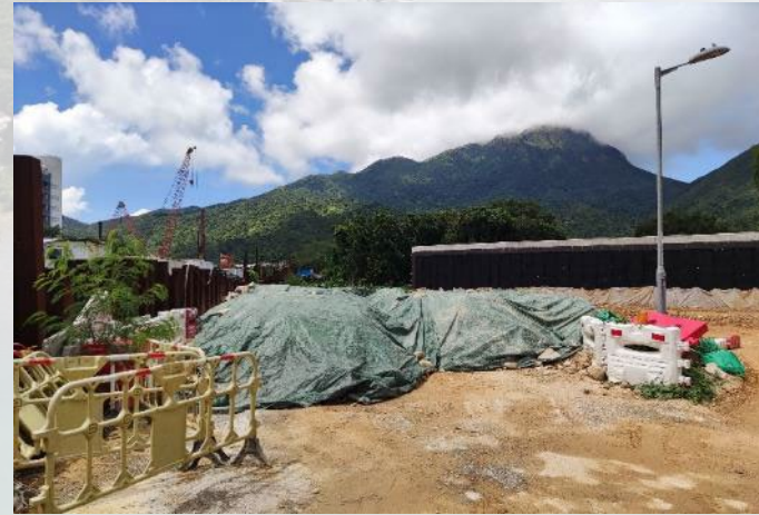
Covering excavated stockpiles by impervious sheeting
