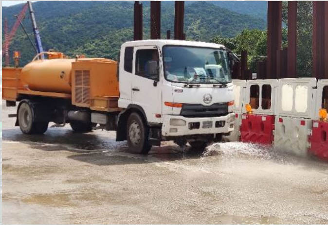
Water spraying by water truck along haul road
