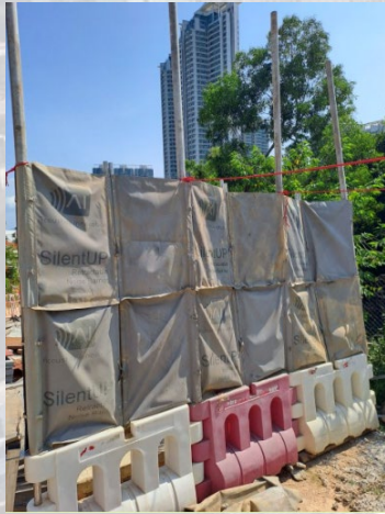
Deployment of noise barrier
